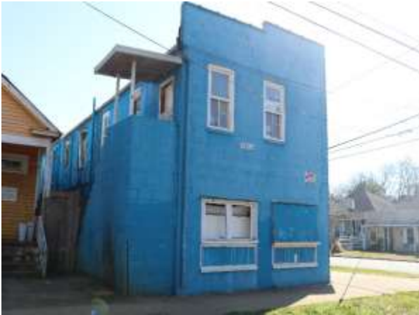
Cozy Corner Pre-Demolition
